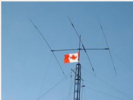
**Antenne Yagi HF tribande**
